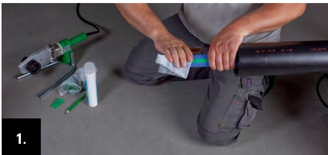
Remove dirt and impurities at the pipe ends. (Note: for the processing of aquatherm blue pipe or ti, also see description on page 22)
