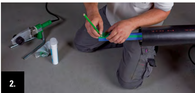
Mark welding depth with the attached blue template and a pencil.
