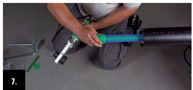
Within the processing time press the welding socket on the pipe end up to the end of the welding depth.
